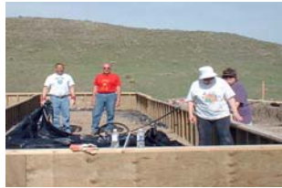
Construction work with 3 supervisors and 1 worker
