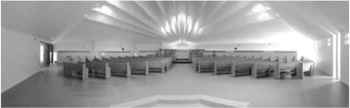
Sanctuary Remodeling in Progress
