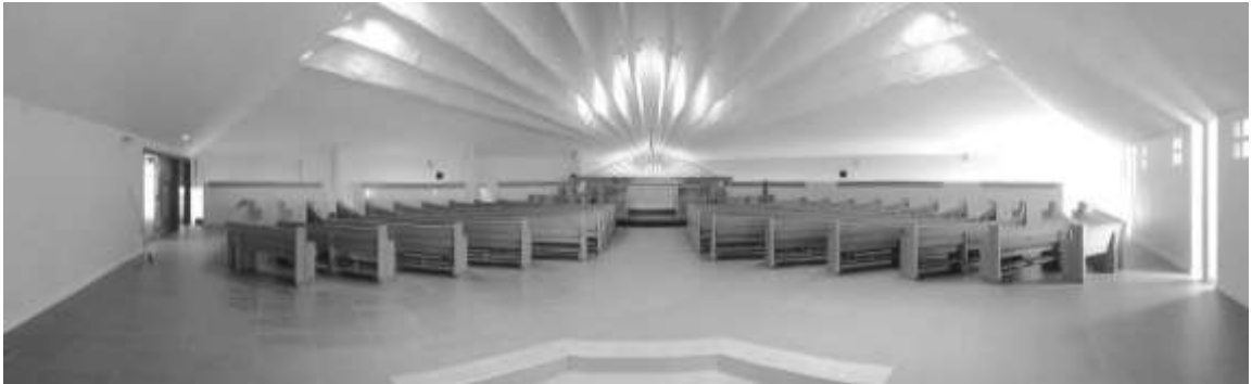
Sanctuary Remodeling in Progress
