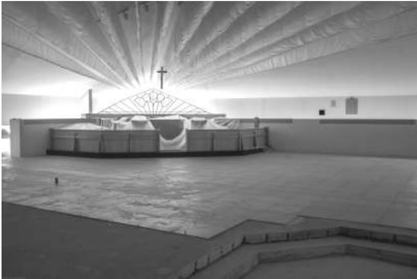
Sanctuary Remodeling in Progress
