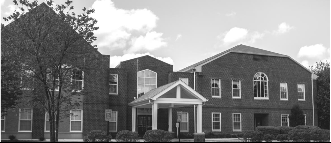
Spring Street Facing Entrance
